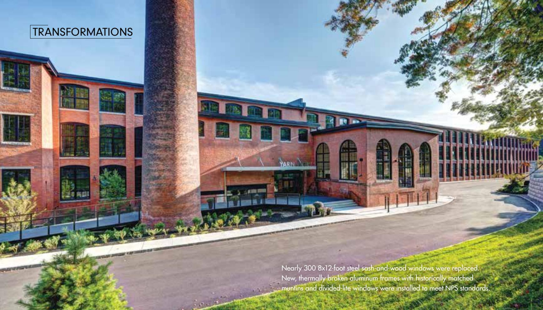
Nearly 300 8x12-foot steel sash-and-wood windows were replaced. New, thermally broken aluminum frames with historically matched muntins and divided-lite windows were installed to meet NPS standards.
